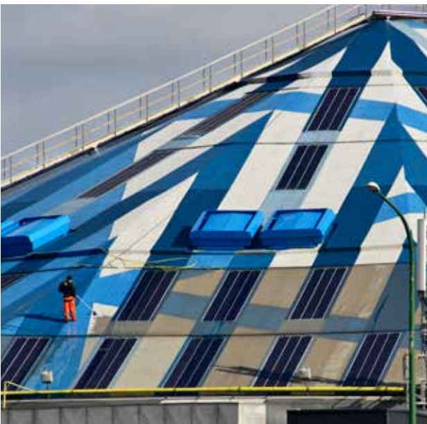
White PVC- P roofing membrane without protective coating
