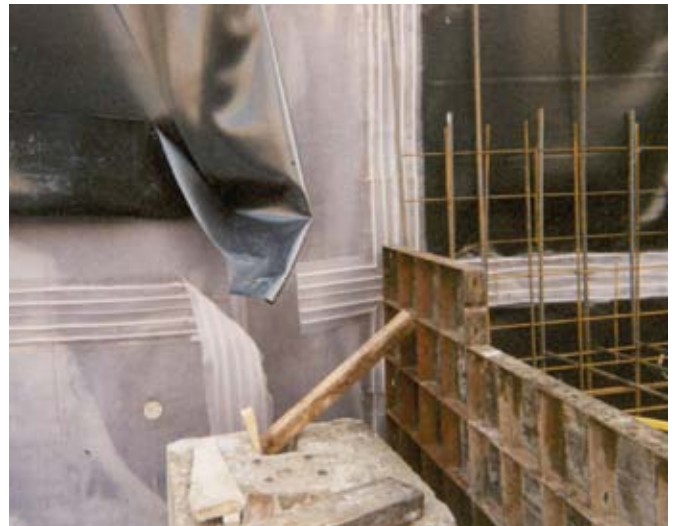
Execution of lining system with water stops
