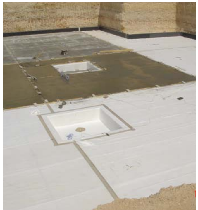
Protected Slab with exposed Water Stops
