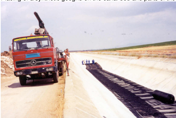
geo-grid as drainage under geocomposite in bed of the canal
