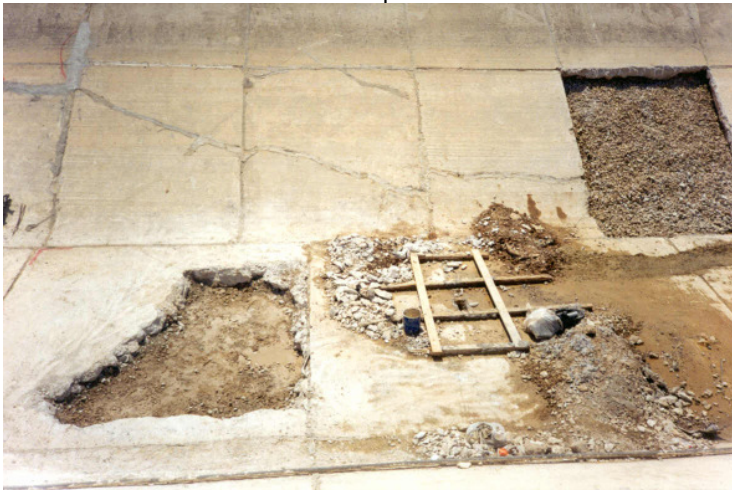
Repair of broken concrete zones.
