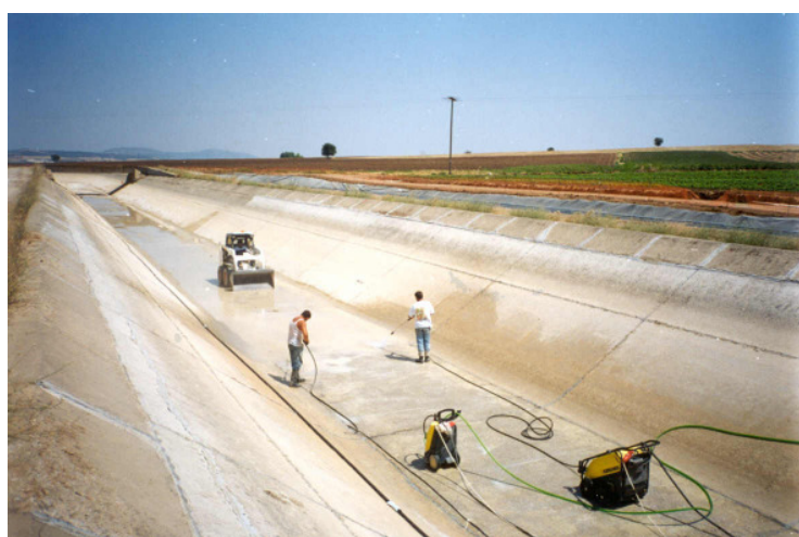
cleaning under high pressure
