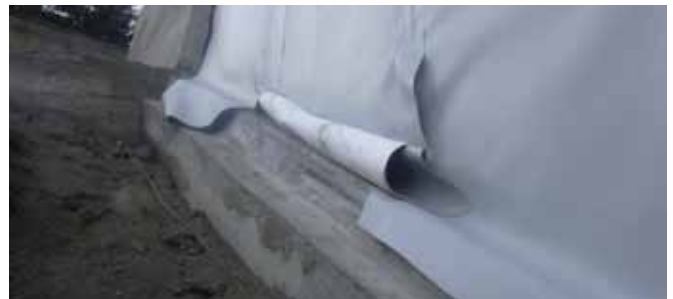
Connection to the concrete structure with the help of loose-fix flange
