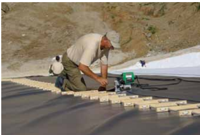
Unrolling and placing of geomembrane
