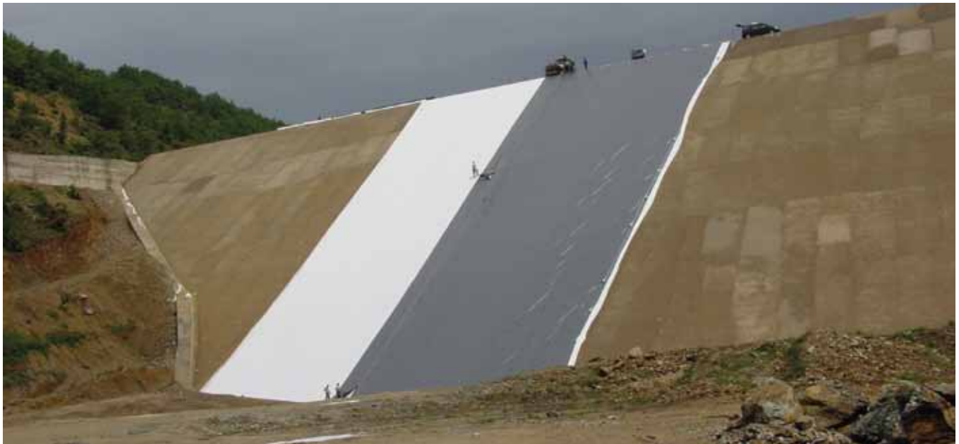
Placing of geotextile
