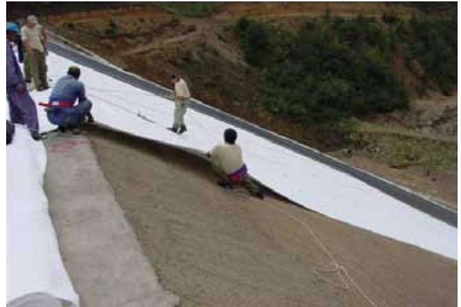
Placing of geotextile
