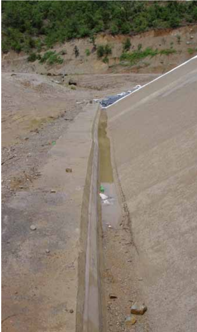
Principle of a flange construction to fix the lining system
