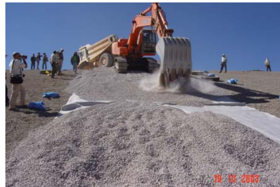
Distribution with excavator
