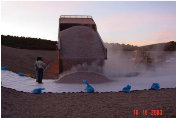
Unloading of protection material with truck
