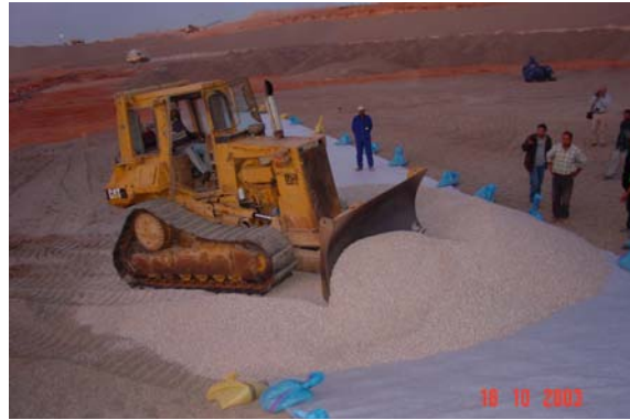
Distribution of material with bulldozer
