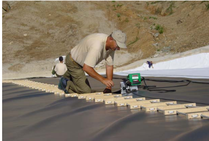
Welding with hot air and double seam
