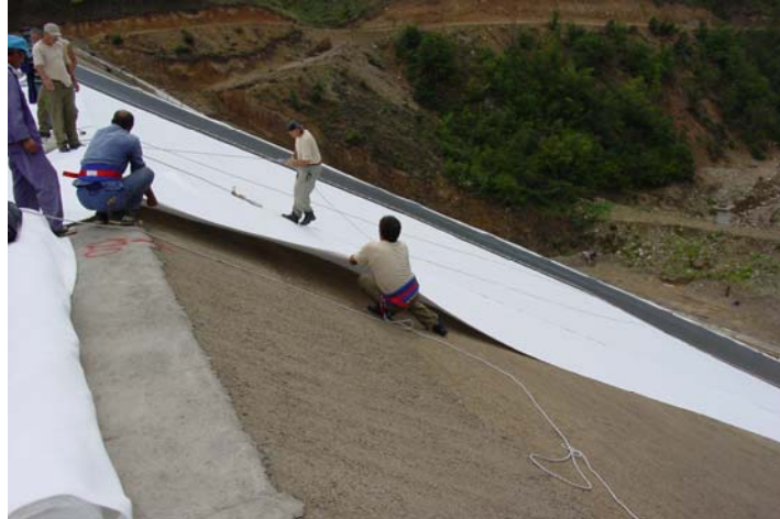
Placing of geotextile
