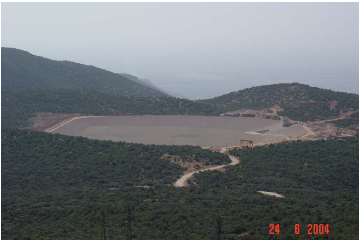
Upper lake for Hydraulic power plant of Afourer in Morocco
