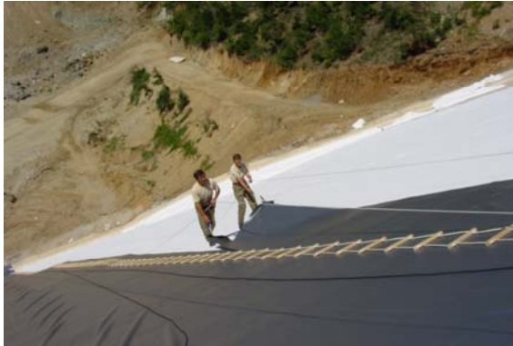
Unrolling and placing of geomembrane
