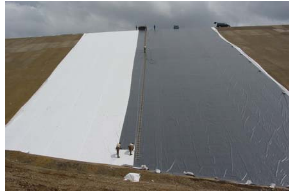
Unrolling and placing of geomembrane
