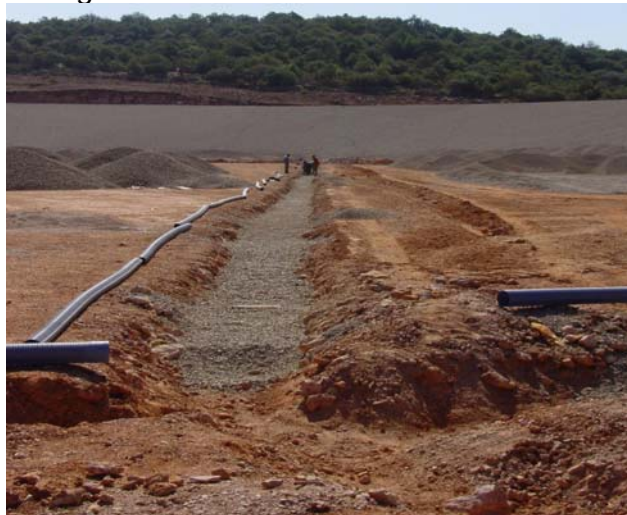
Drainage pipes under waterproofing
