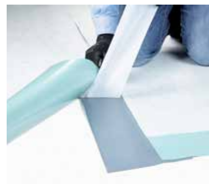
Sealing by butyl tape RENOLIT ALKORPRO BAND .
