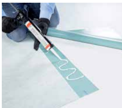
Sealing by mastic glue RENOLIT CEM 805 .
